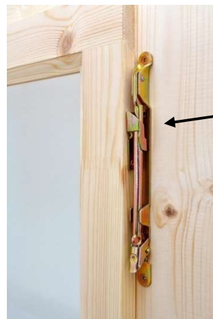
latch unlocked allows window to 'tilt' open
