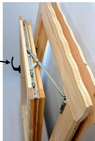
Double glazed window with 'tilt' and 'turn' action within handle
