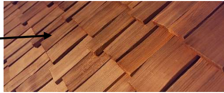
Cedar Shingle Roofing
